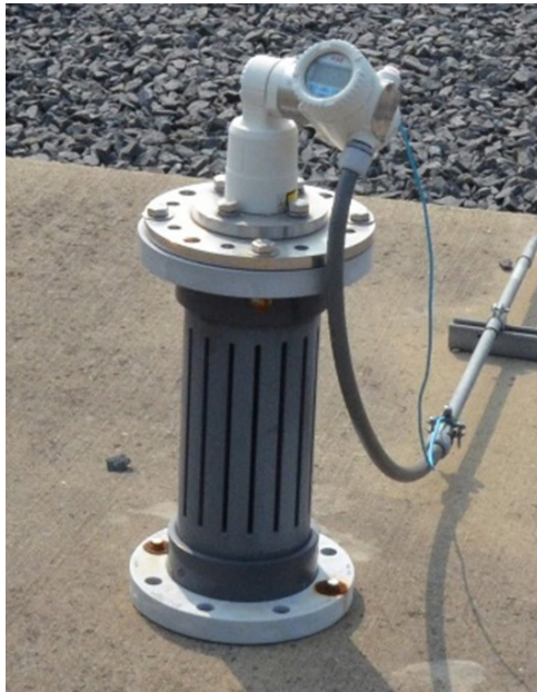
Top of 60 ft Utility Shaft
